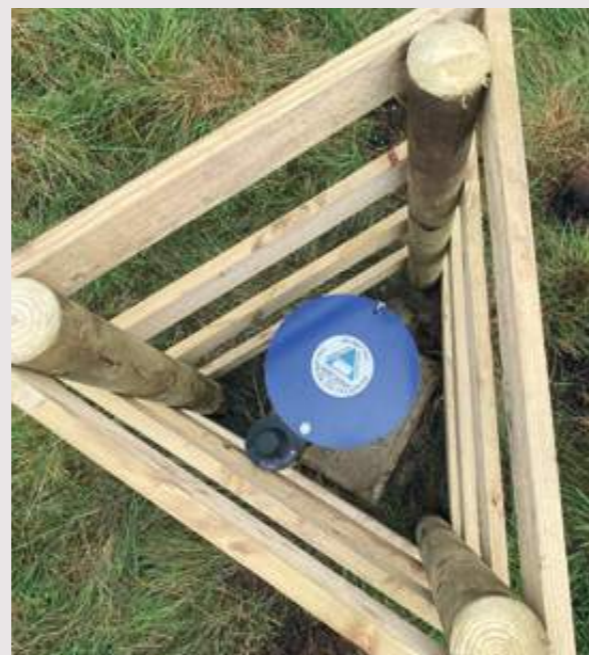
Typical groundwater monitoring well
