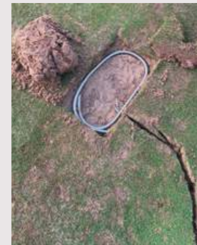
Installing pH sensors
